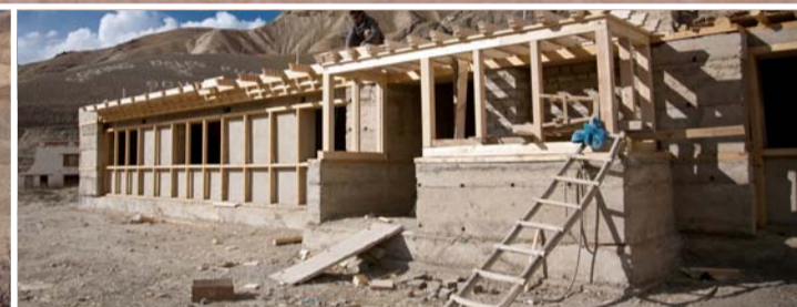
... construction already started
