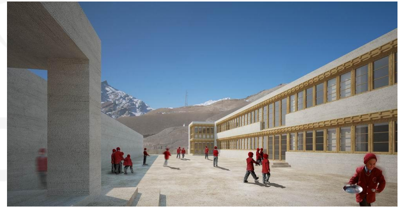
2012 - 2014 : First block of classrooms
