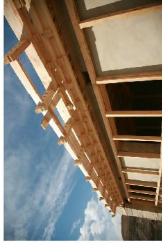
IMPROVED TRADITIONAL LADAKHI WINDOW DECORATION TO WORK FOR PASSIVE SOLAR BUILDINGS PROTECTING AGAINST OVERHEATING
