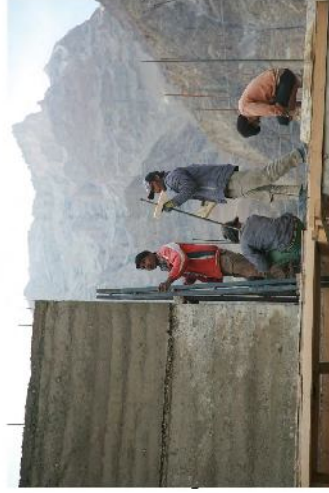
IMPROVED TRADITIONAL LADAKHI RAMMED EARTH WALL
