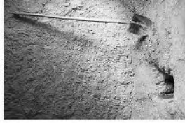
TRADITIONAL LADAKHI RAMMED EARTH WALL
