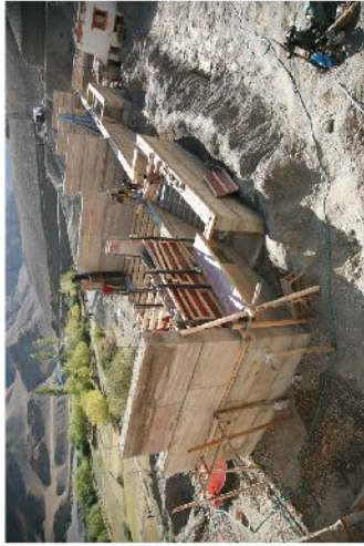
IMPROVED TRADITIONAL LADAKHI RAMMED EARTH WALL
