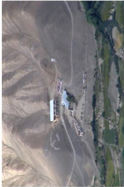
OVERALL VIEW OF THE CURRENT SCHOOL
