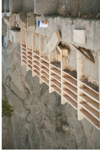
IMPROVED TRADITIONAL LADAKHI WINDOW DECORATION TO WORK FOR PASSIVE SOLAR BUILDINGS PROTECTING AGAINST OVERHEATING
